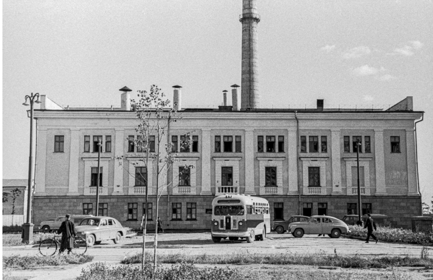
Figure 3: Obninsk Power Plant
